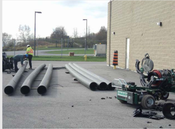
New HDPE pipe to be Butt-Fused for Suction and Discharge
