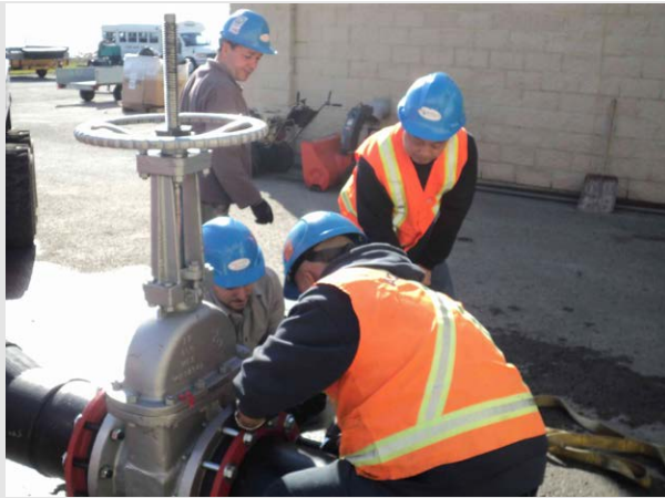
Aquatech team bolting the 12" pipe to gate valve
